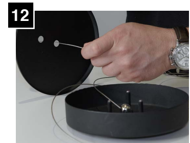
12 Feed aircraft cable through backside center hole of canopy cover.
